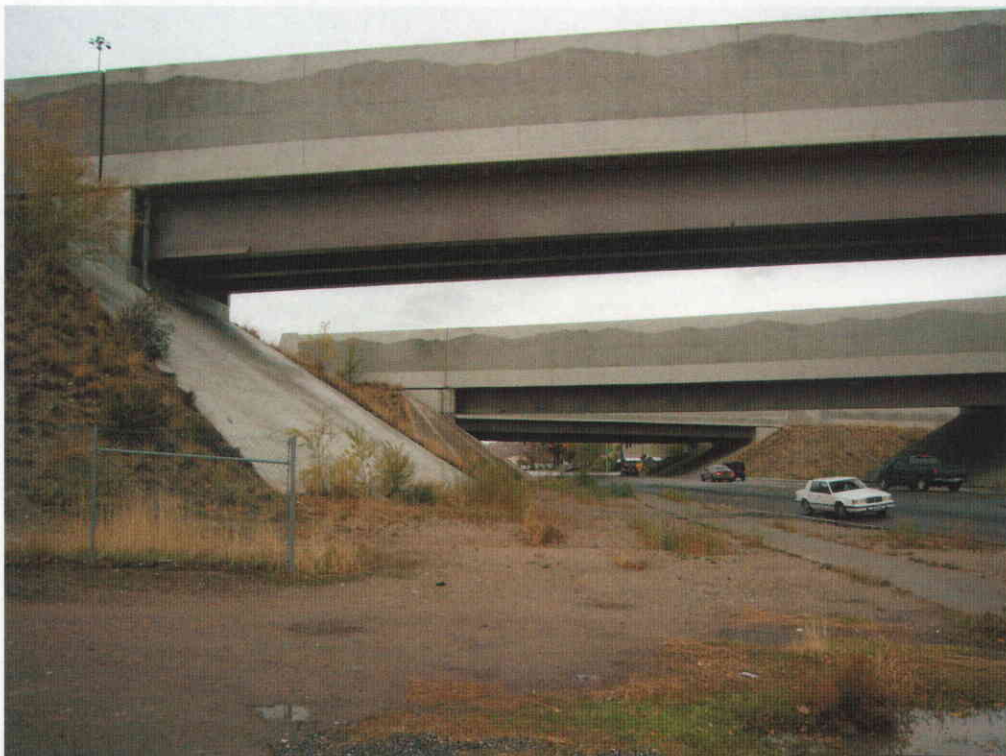
Looking north on 900 West from approximate location of driveway
